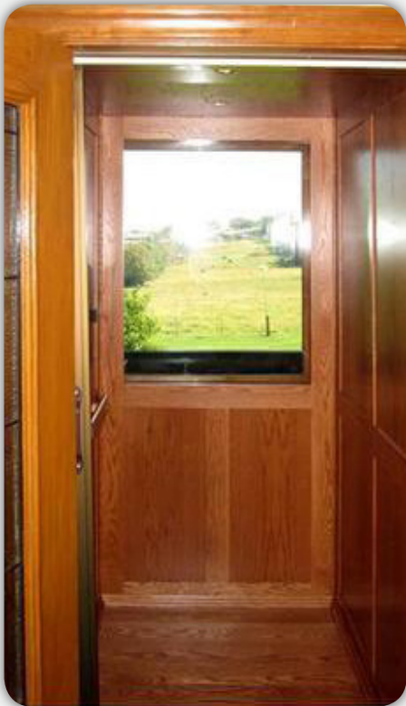
Residential elevator with Shaker panels and an upper window
